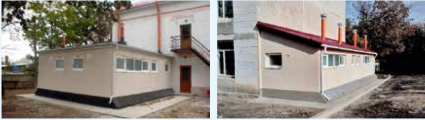
Figure 3: Examples of ecosan toilet blocks attached to existing school buildings Source: Skat Foundation (ApaSan)
